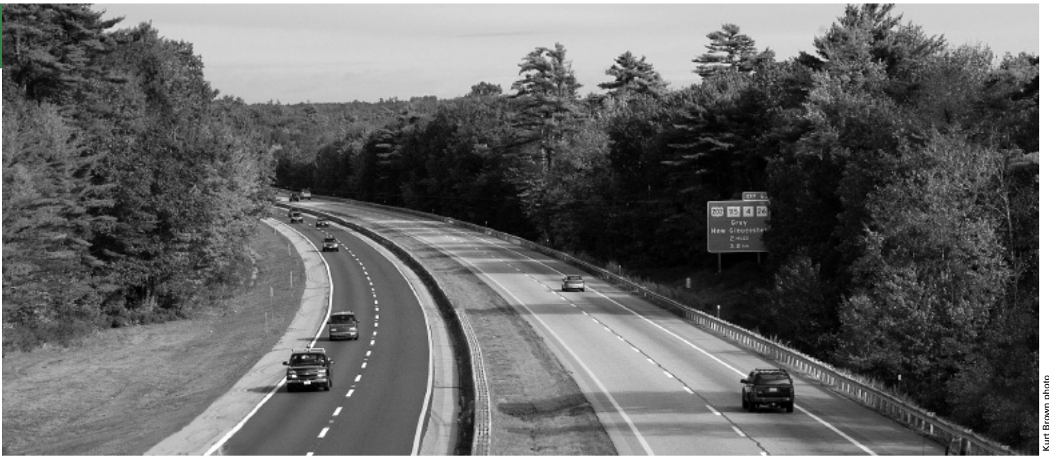
Major paving projects were completed in 2008, including 7.4 miles of southbound lanes between Cumberland and Gray.
