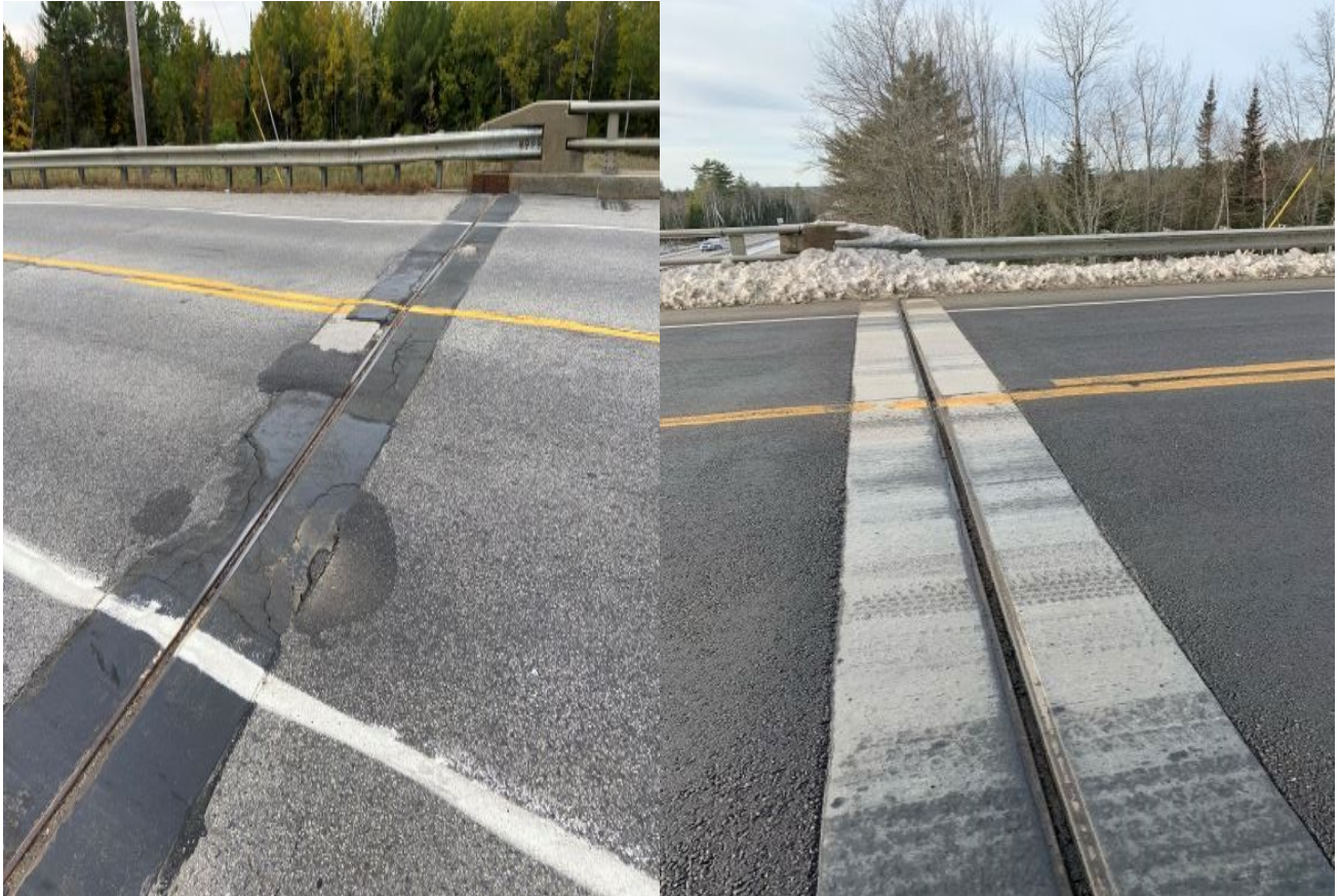
Kitty Hawk Road Bridge western joint, looking south: before and after.
