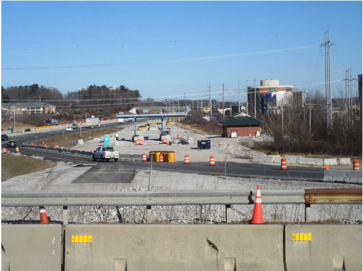
Northbound Toll Plaza
