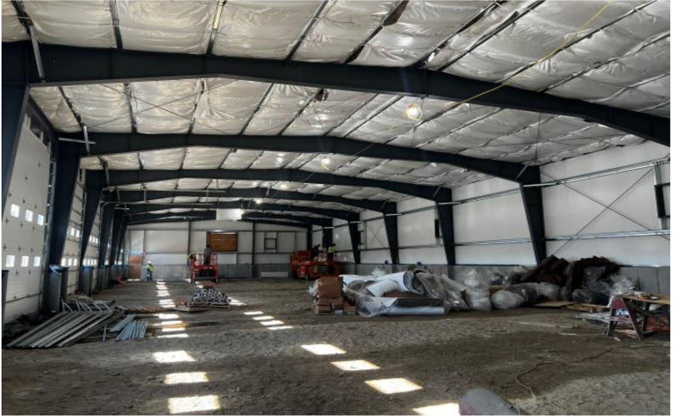
Looking west inside the new 8 bay garage. Crews are working on the ceiling insulation.
