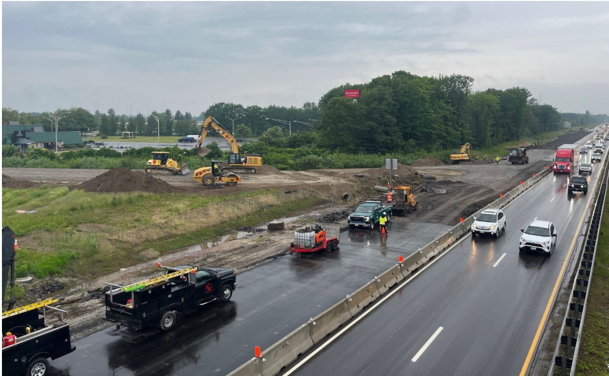
Excavating and fine grading during exit 48 southbound off ramp closure.
