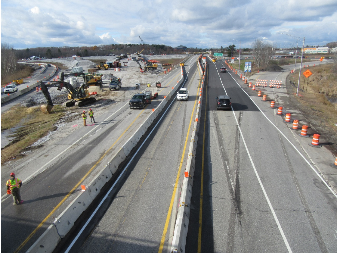
Exit 45 Interchange looking toward the Turnpike after entering thru Toll Plaza
