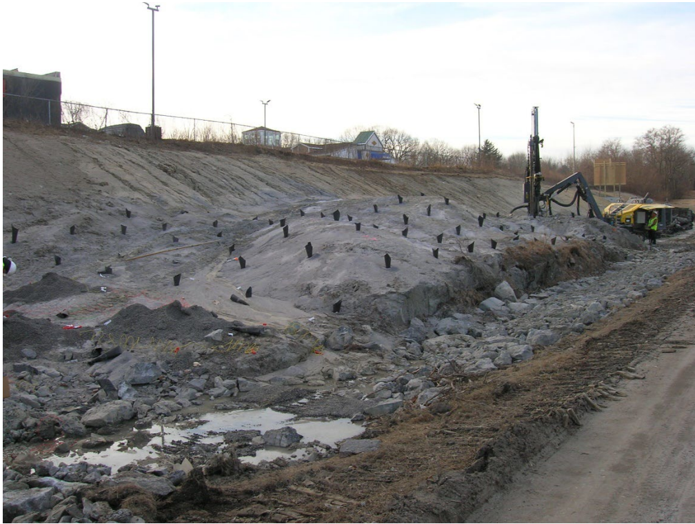
Drilling holes for ledge blasting at Brighton Avenue
