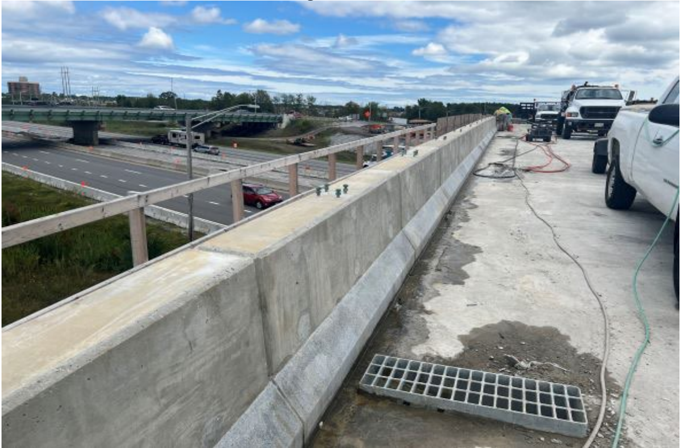
Looking east at crews sealing construction joints on the approach slab
