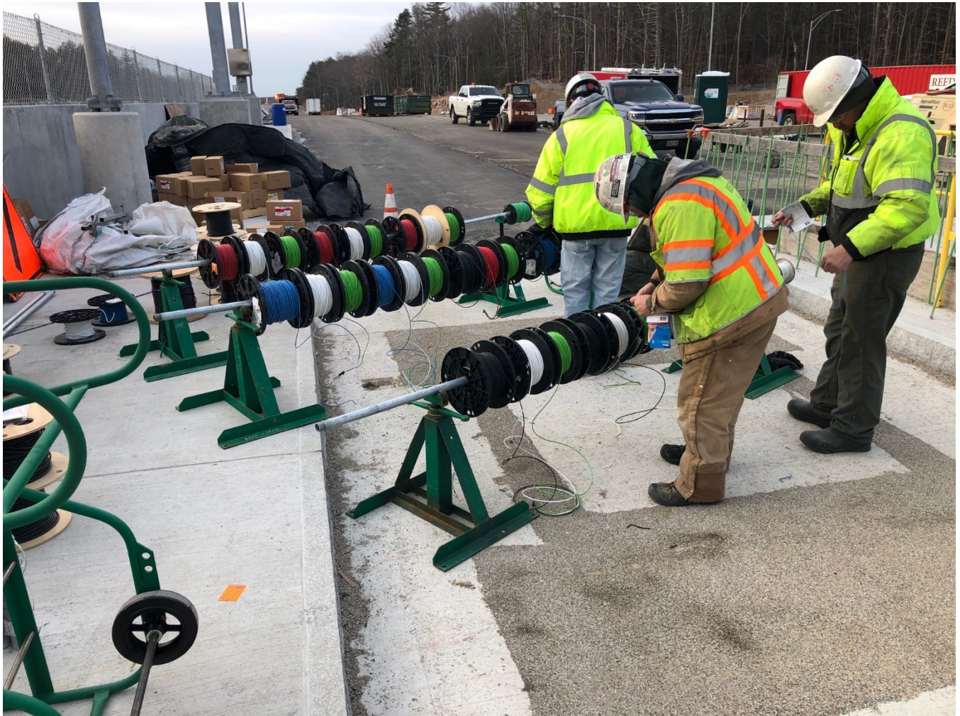
Electricians preparing wire bundles to pull through conduits
