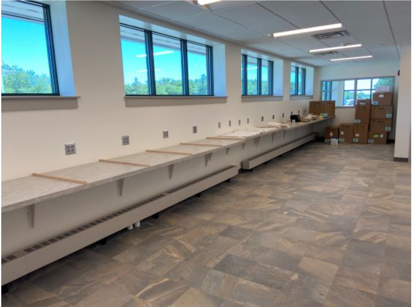
Toll collector work stations are nearly complete inside the new building.
