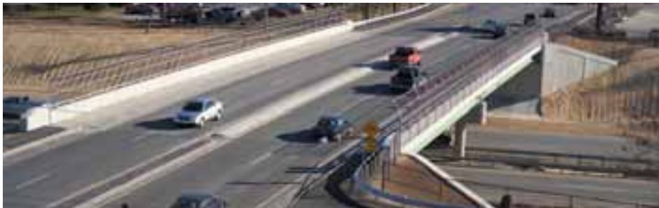
The Authority successfully completed two major bridge projects, including Brighton Avenue Bridge (above) which carries 35,000 vehicles a day.
