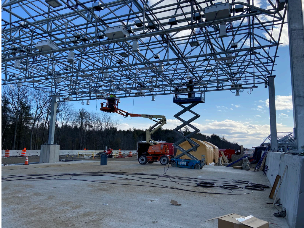
Reed & Reed electricians pulling data lines to the ORT structure.
