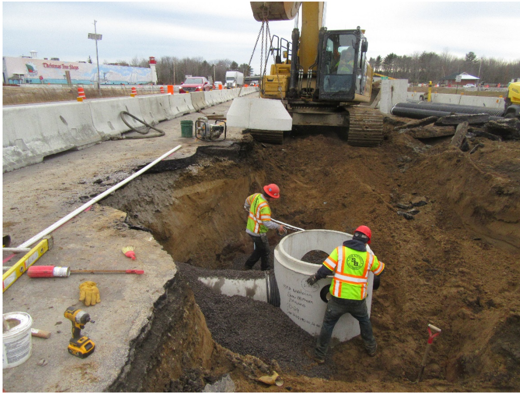
Installing catch basin base in median
