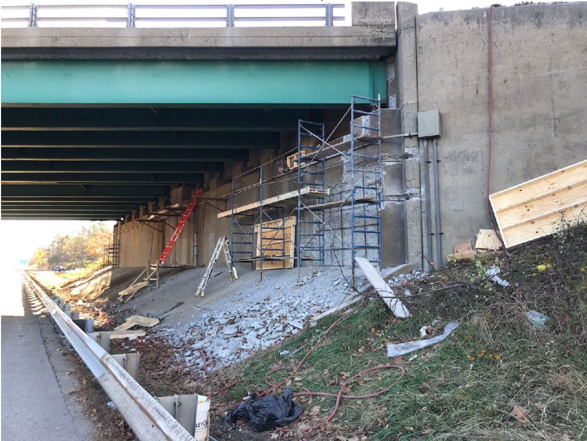
Route 236 bridge looking at the west abutment: crews performing concrete repairs.
