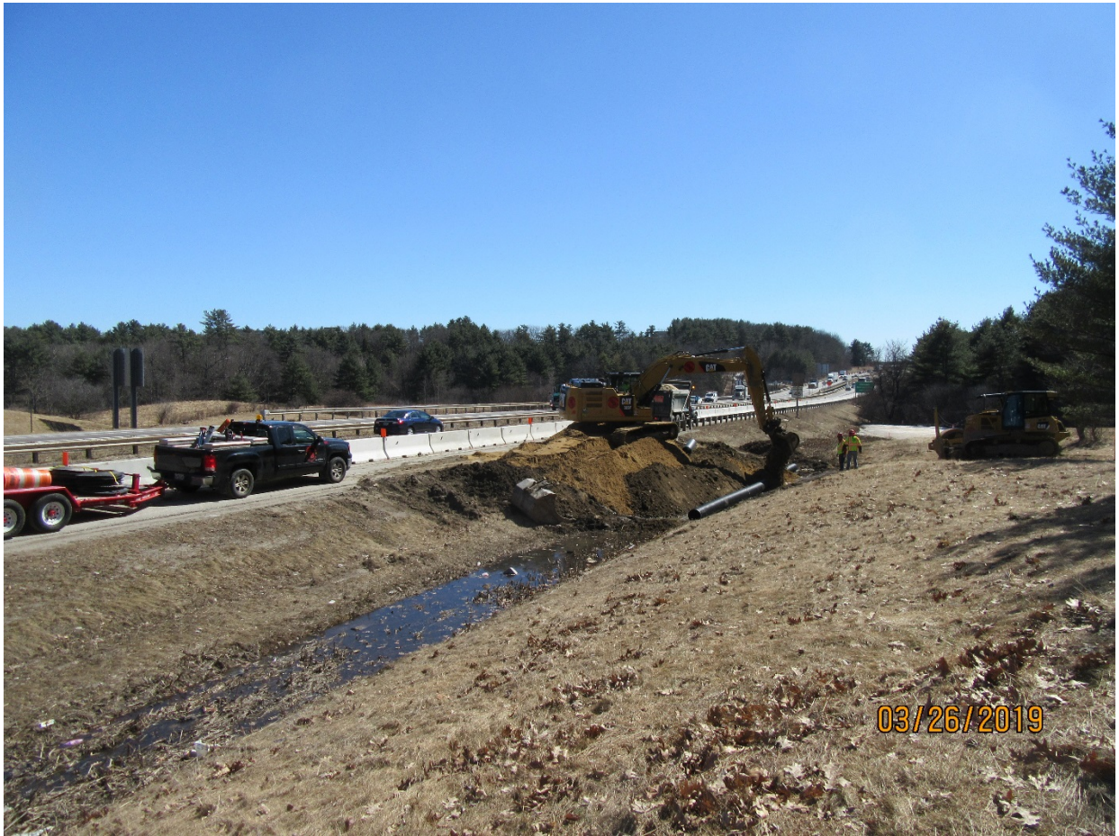
Work at Stroudwater Bridge Southbound – installing culvert for temporary road
