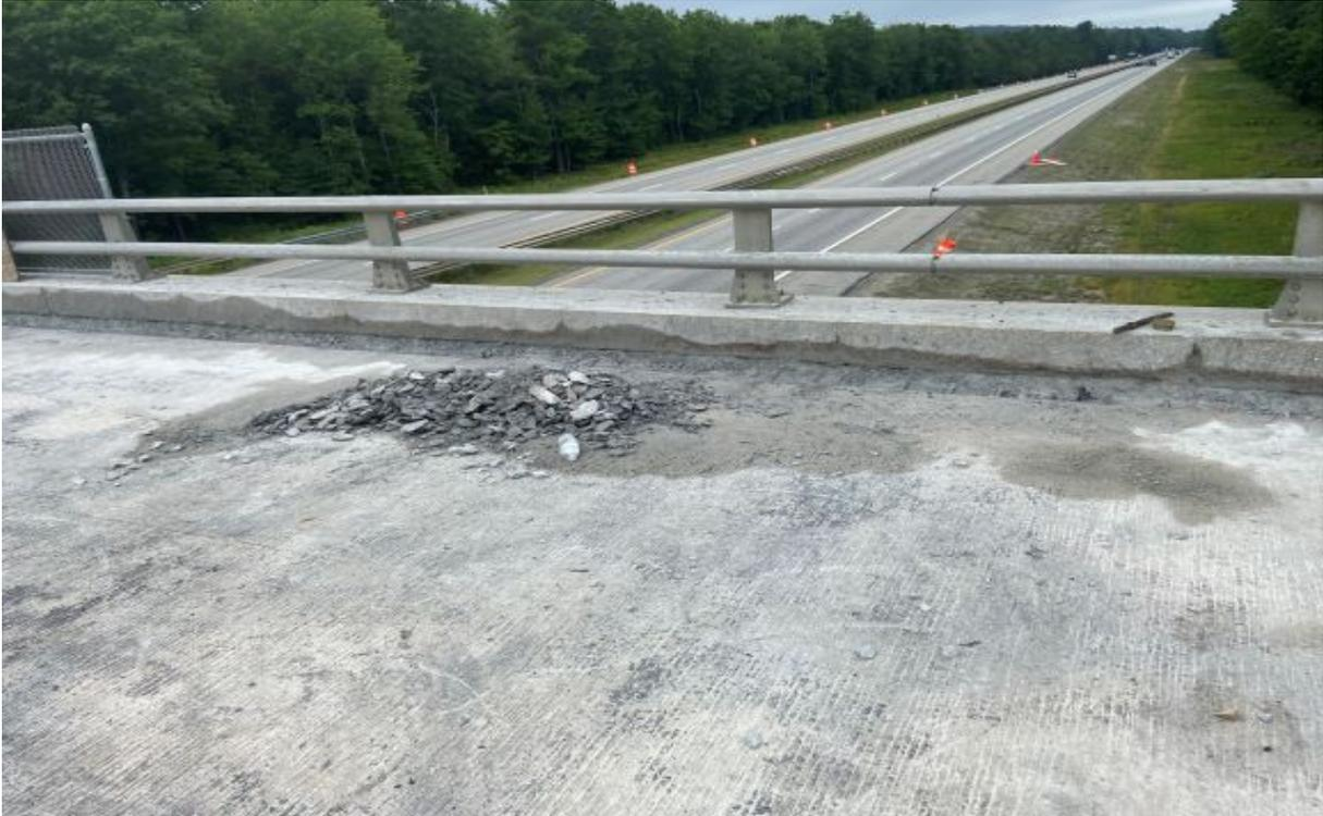
Bennett Road looking north. The concrete deck was in poor condition along the gutter lines.
