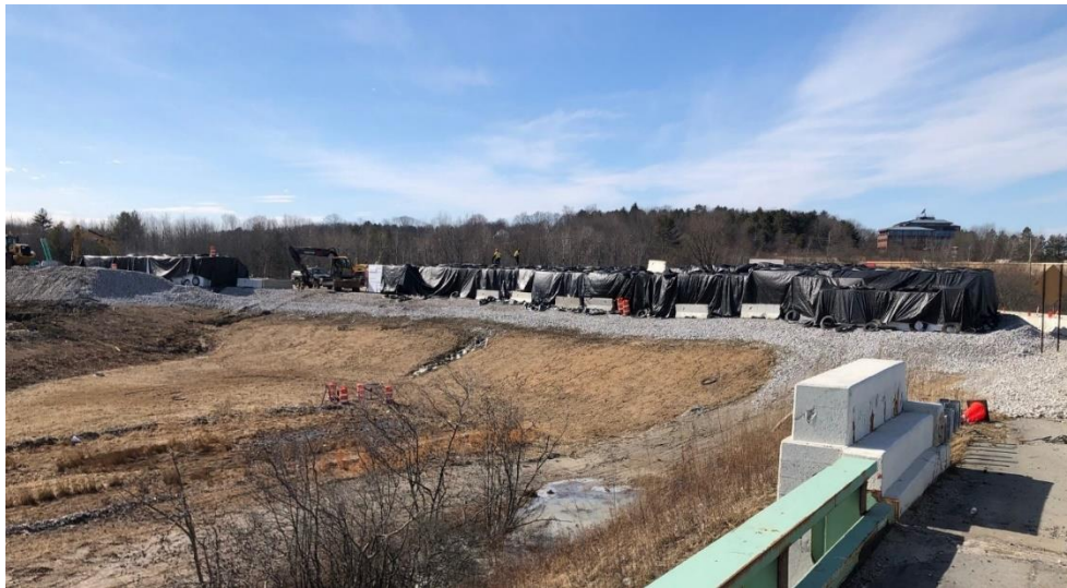
Stacked lightweight geofabric blocks
