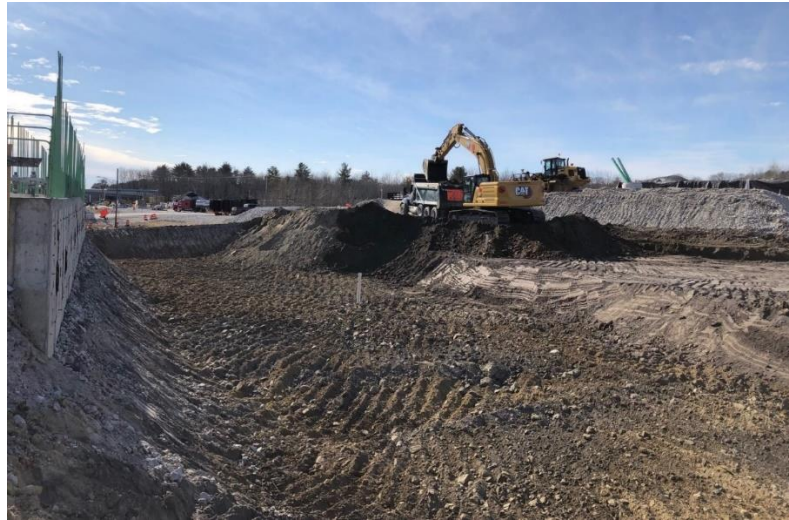
Excavating bridge approach
