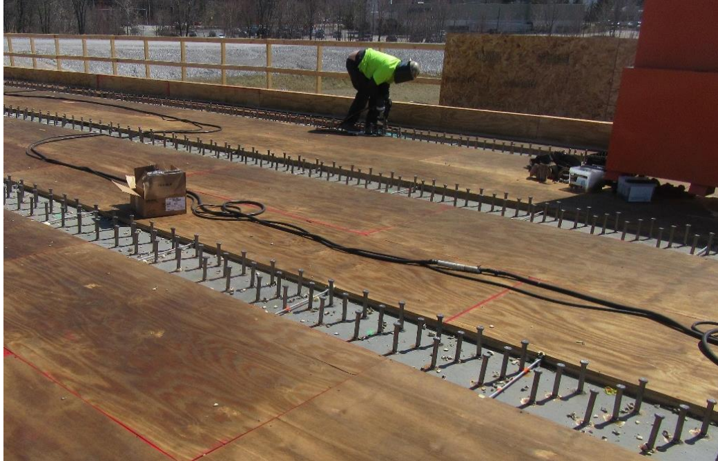
Manually welding on the shear stud connectors, there are over 3,000 connectors
