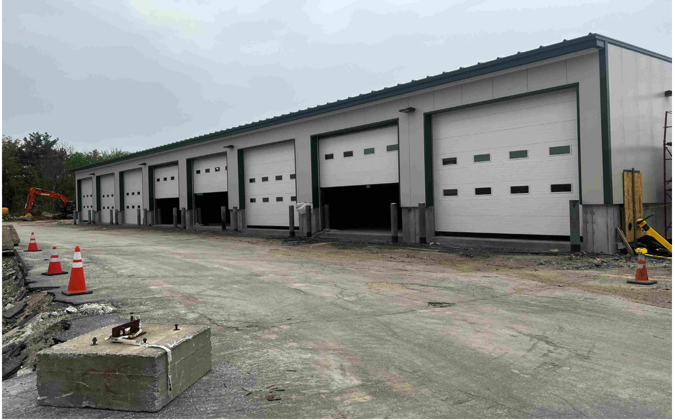
The building with the new doors, bollards, and exterior lighting.
