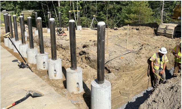
A row of bollards that will protect the future propane tanks needed to heat the new 6-bay garage.
