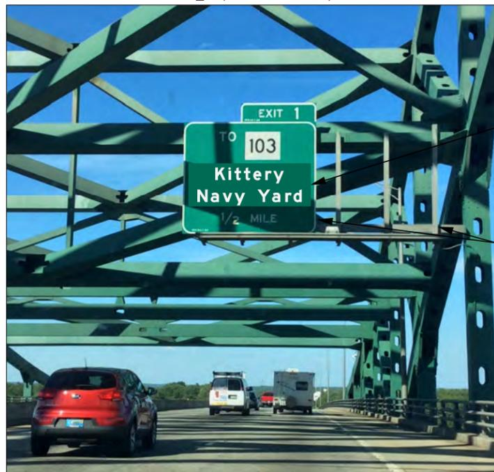
INSTALL NEW SHEET ALUMINUM OVERLAY OL-1 ON EXISTING SIGN
