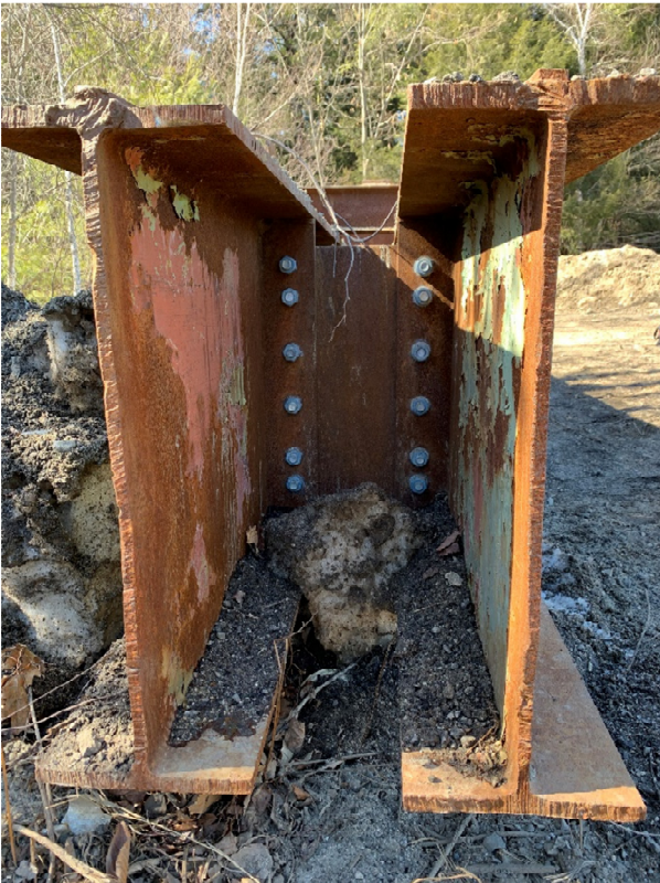
Photo 9 – End View of the MTA’s Strongback
