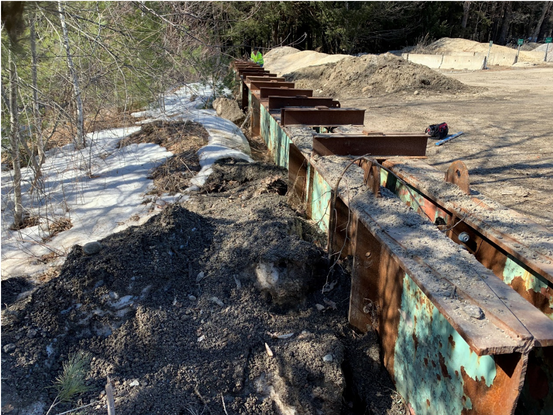
Photo 10 – Photo of MTA Strongback Showing Lifting Devices and Stiffeners
