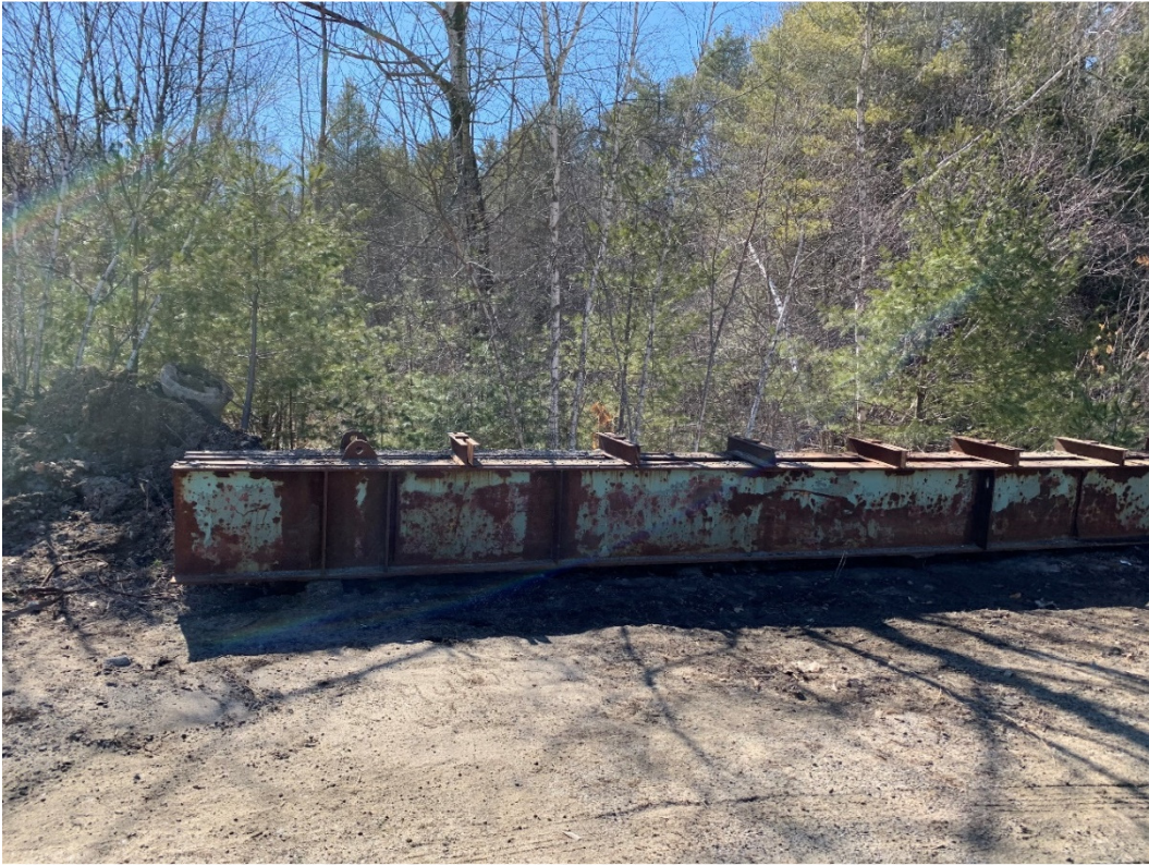
Photo 8 – Elevation View of the MTA’s Strongback
