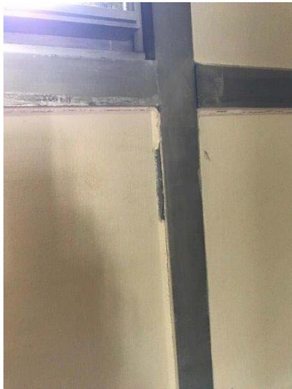
Picture 5: window caulking that tested positive for asbestos, which is attached to the transter panels
