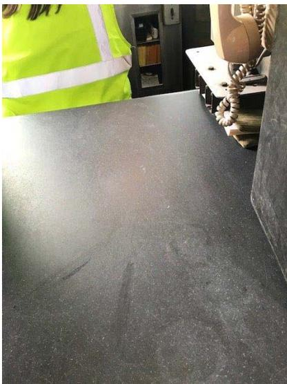
Picture 3: toll booth lab tops are assumed to be asbestos based on previous testing of the materials
