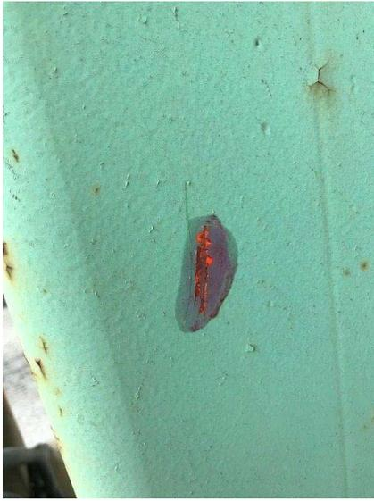
Picture 4: structural steel supports positive for lead based paints
