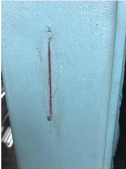
Picture 1: Structural steel supports tested positive for lead paint
