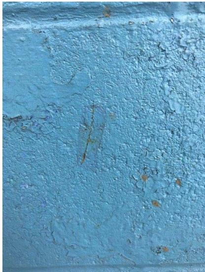
Picture 2: painted cement block at tool booths tested negative for lead paint
