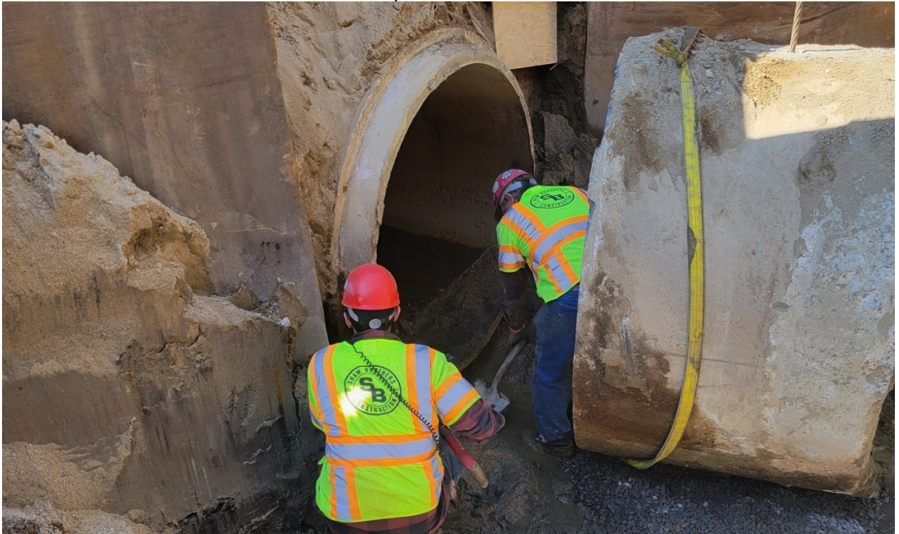
Extension of a 60 inch culvert crossing.
