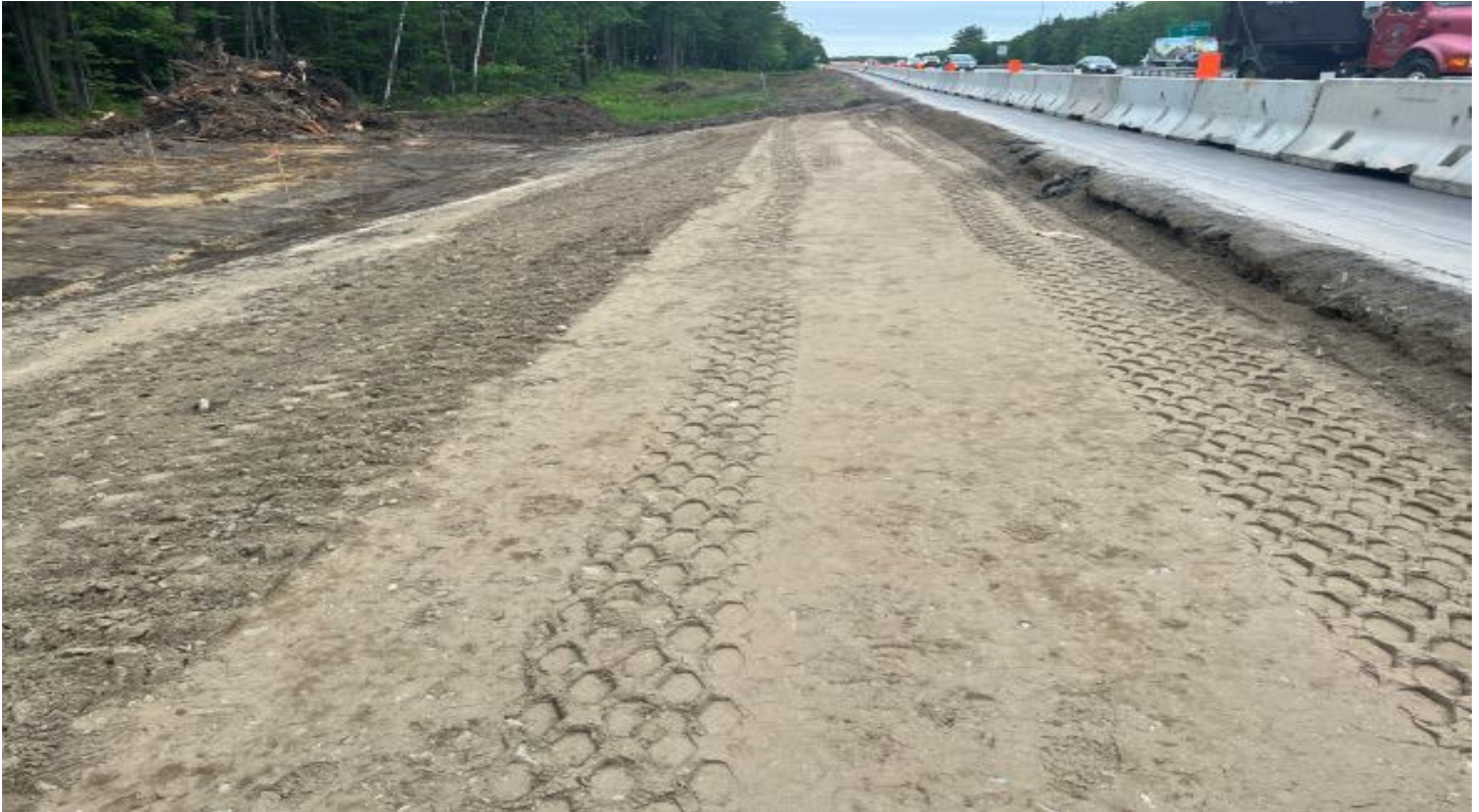
Looking south at the recently widened northbound Exit 36 acceleration lane.
