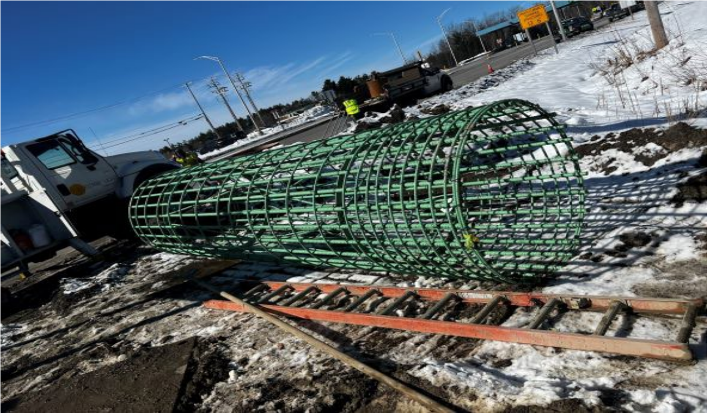
The rebar cage for the mast arm foundation at Exit 42.
