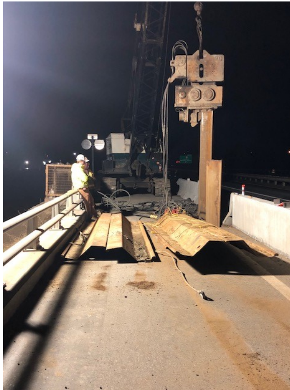
Driving temporary earth support system at MCRR
