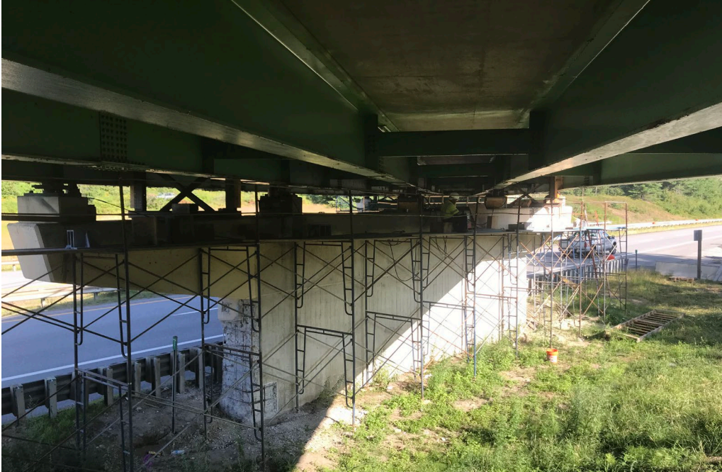
Shaker Road Bridge Jacking and concrete repairs.
