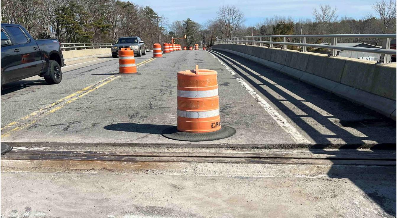
Looking east, crews have removed and prepped the existing joints for repairs. They will return and repave the bridge at a later date
