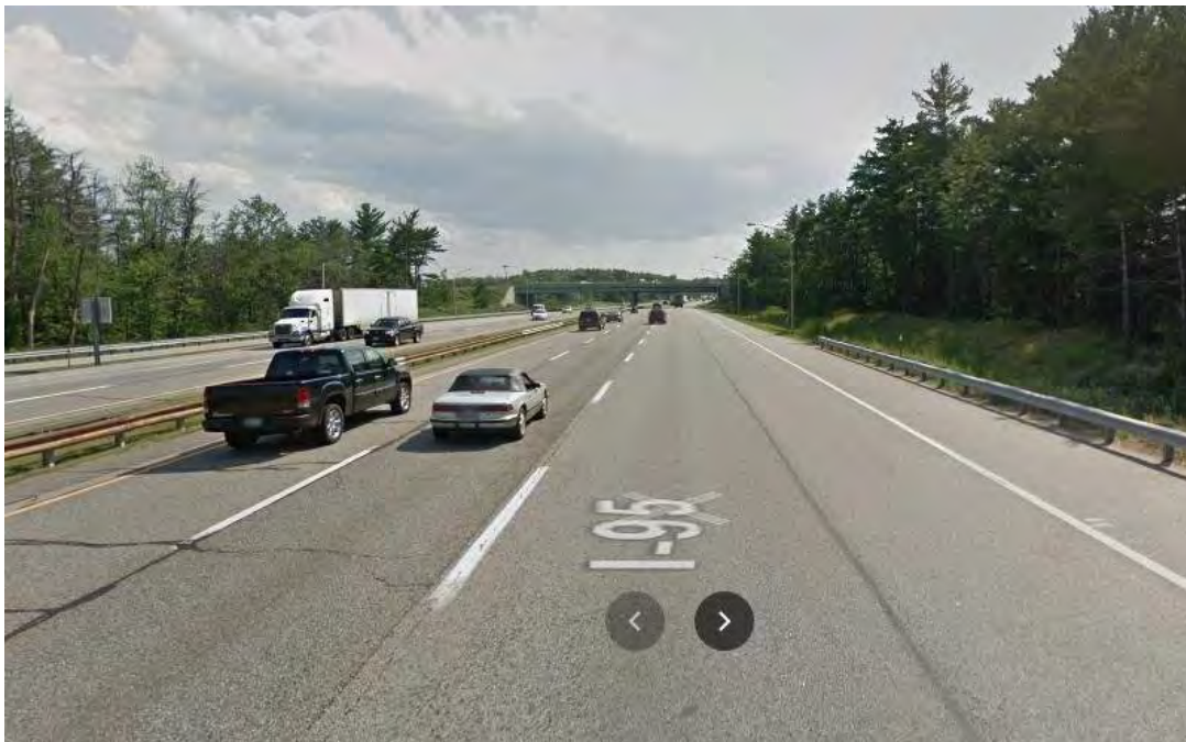
Photo 2: Segment after Exit 32 SB On Ramp (2011)
