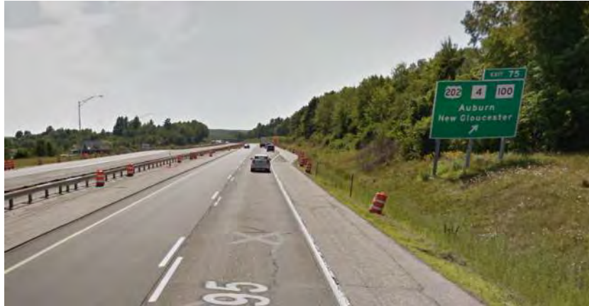
Photo 1: I-95 SB North of Exit 75 Interchange (2018)
