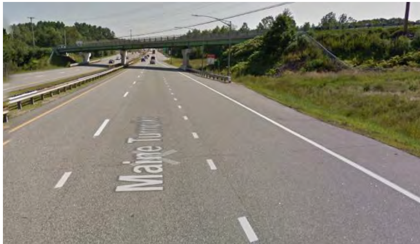
Photo 1: Just South of Exit 53 Southbound On Ramp
