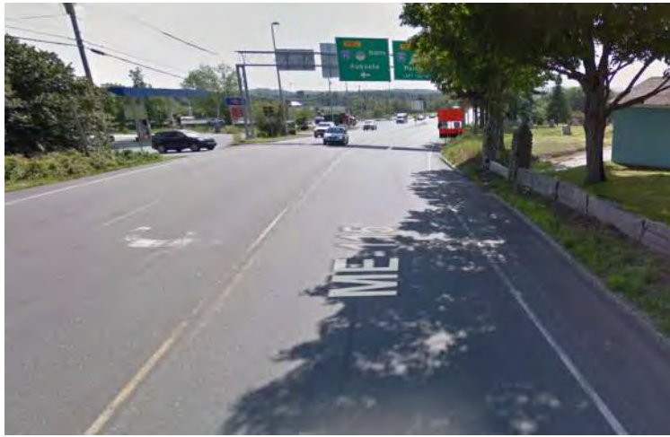
Photo 1: NB Ramps Intersection WB Approach (2018)
