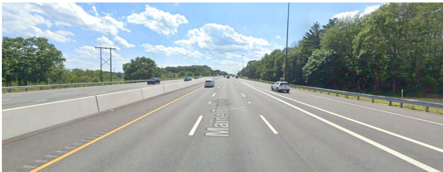
Photo 1: Exit 2 SB On Ramp Merge Point (July 2022)
