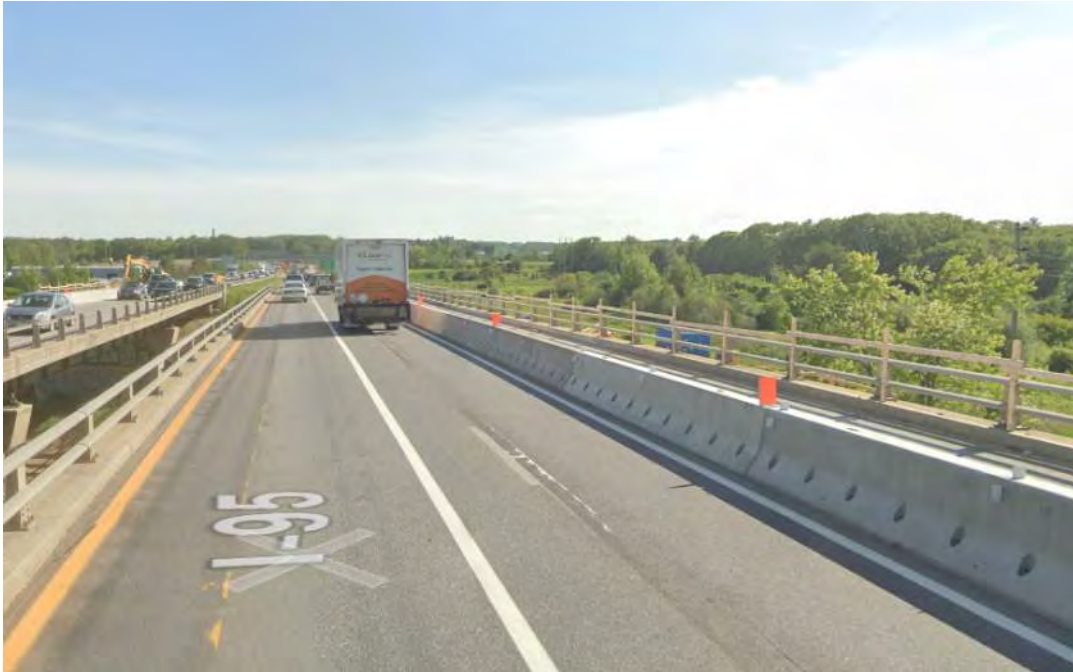
Photo 1: I-95 SB Just North of Exit 47 Off Ramp (2019)
