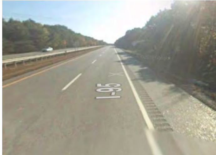
Photo 3: North of SB Toll Plaza (2008)
