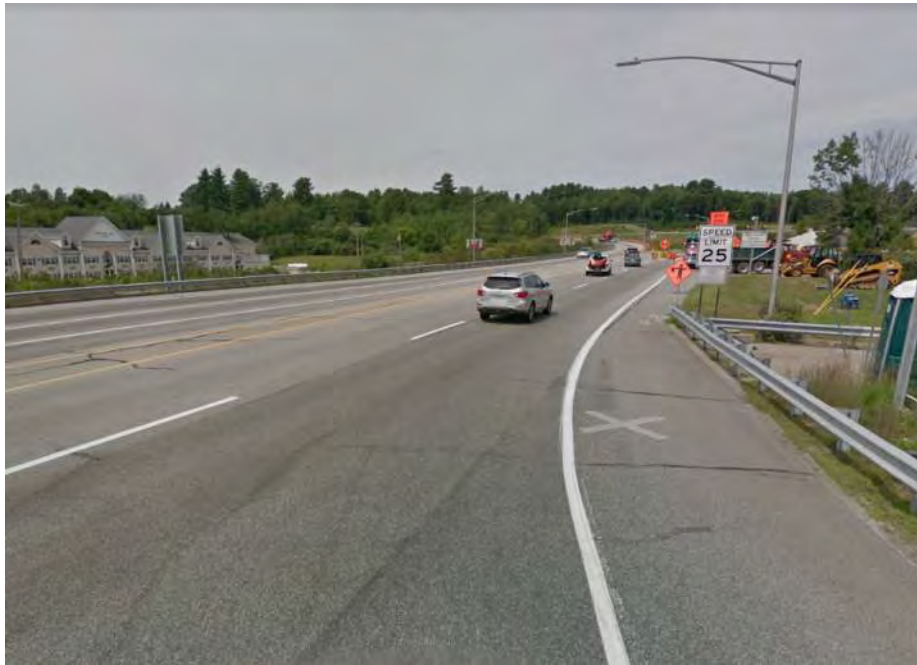
Photo 1: Exit 75 Ramps Weave (2018)
