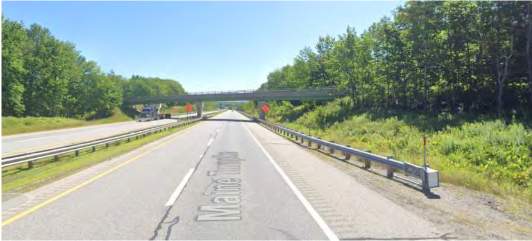
Photo 1: NB Segment Near Academy Road (2022)
