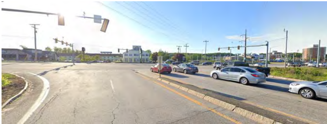
Photo 3: Exit 45 On Ramps Intersection (2019)
