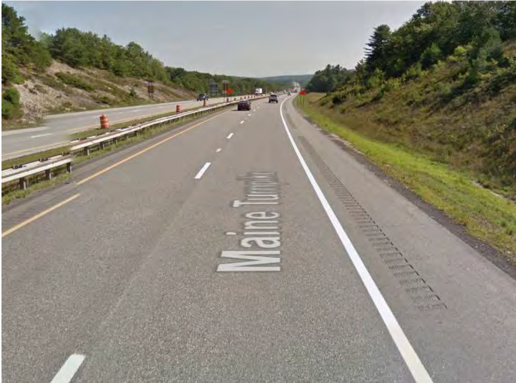
Photo 2: SB South of Upper Blackstrap Road (2018)
