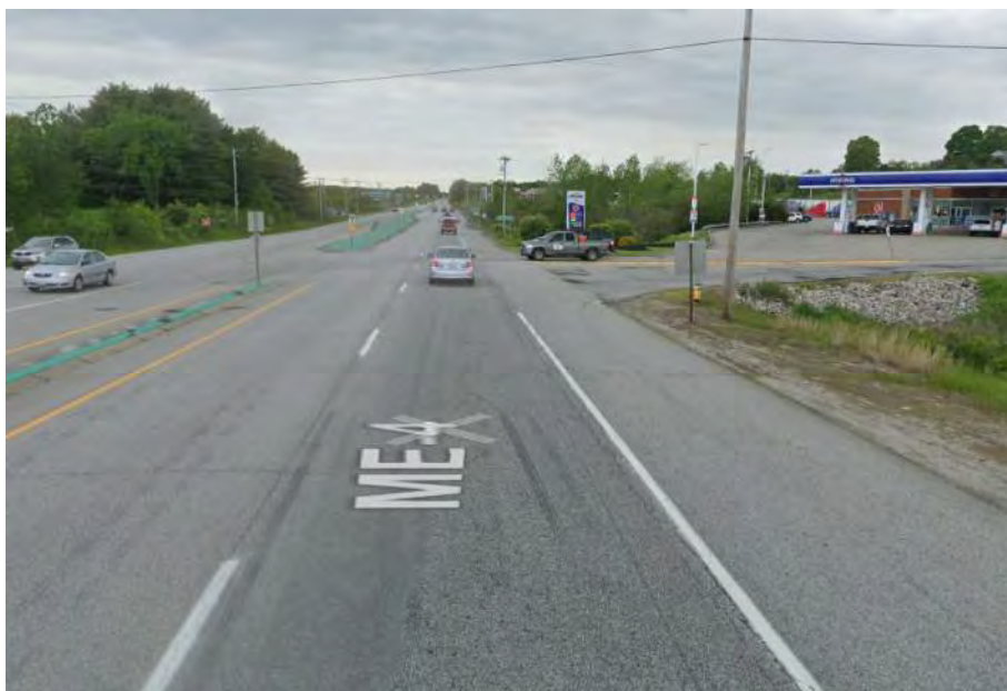
Photo 3: Washington Street at Irving Drive (2019)
