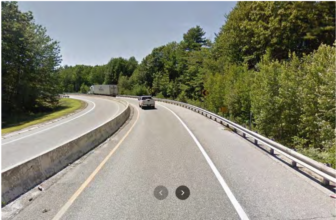
Photo 1: Exit 36 SB Off Ramp
