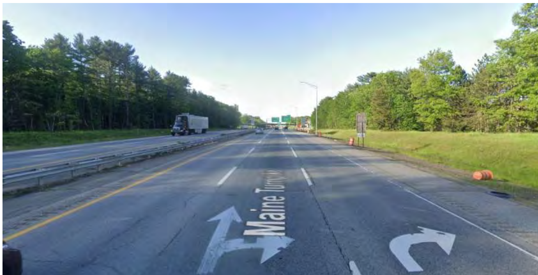
Photo 2: Just South of the Exit 44 NB Off Ramp
