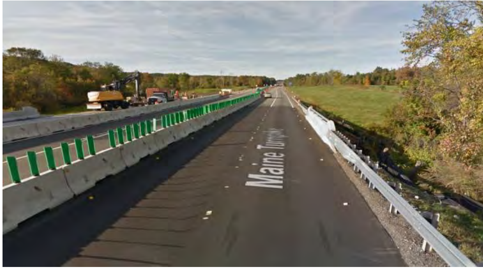
Photo 1: NB Just North of Hurricane Road (2015)
