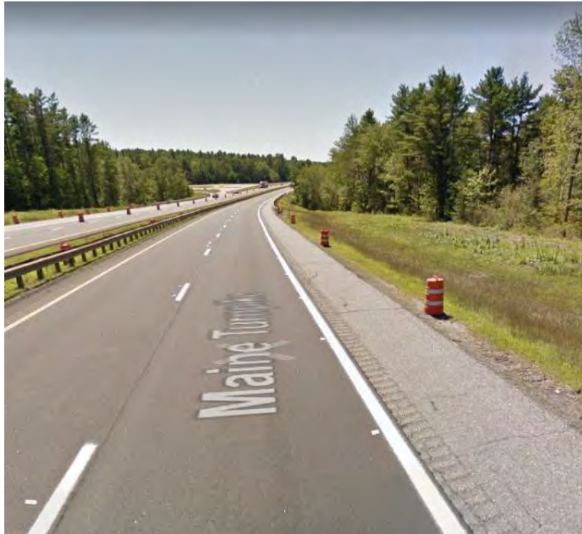
Photo 5: SB Segment Near Stevenstown Road
