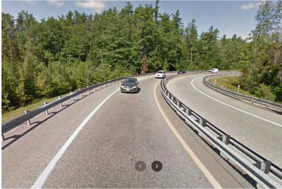
Photo 5: Exit 32 SB Off Ramp
