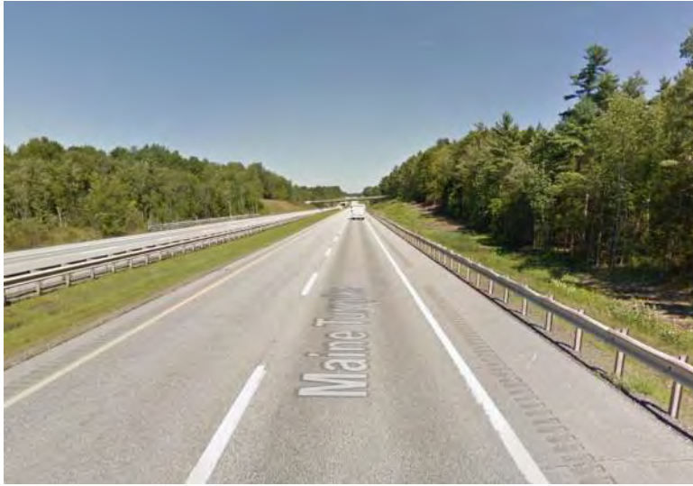
Photo 3: NB Segment Near Stevenstown Road
