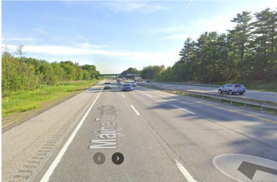
Photo 2: Just Prior to Exit 42 NB Off Ramp
