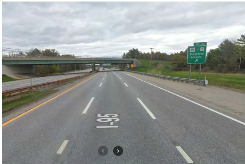
Photo 1: Exit 32 NB Off Ramp Approach (2019)
