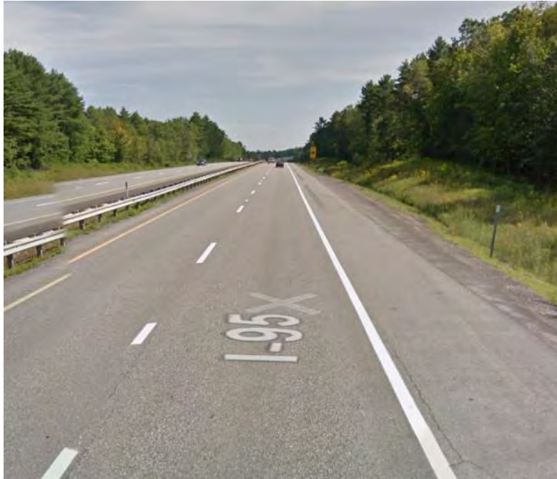
Photo 2: SB South of Exit 63 On Ramp (2018)
