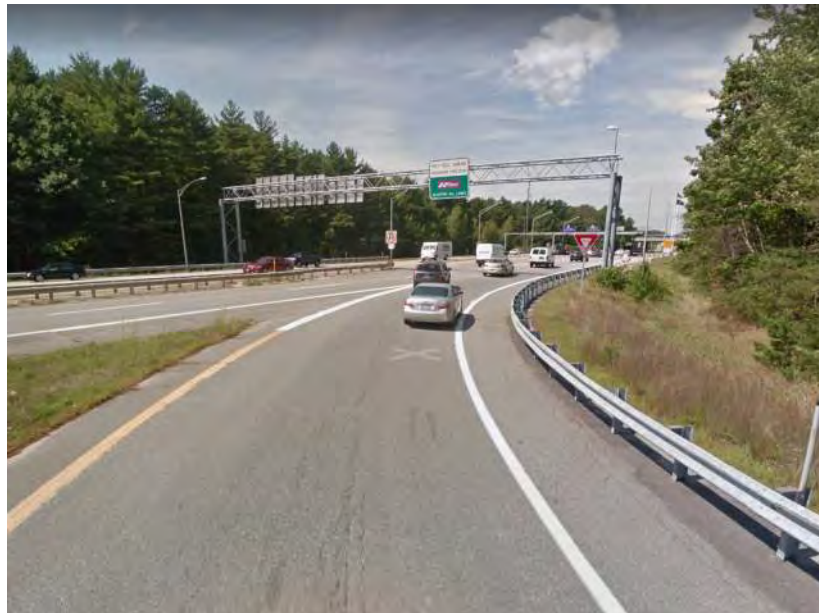
Photo 2: Route 703 Merge with Exit 45 On Ramps (2016)
