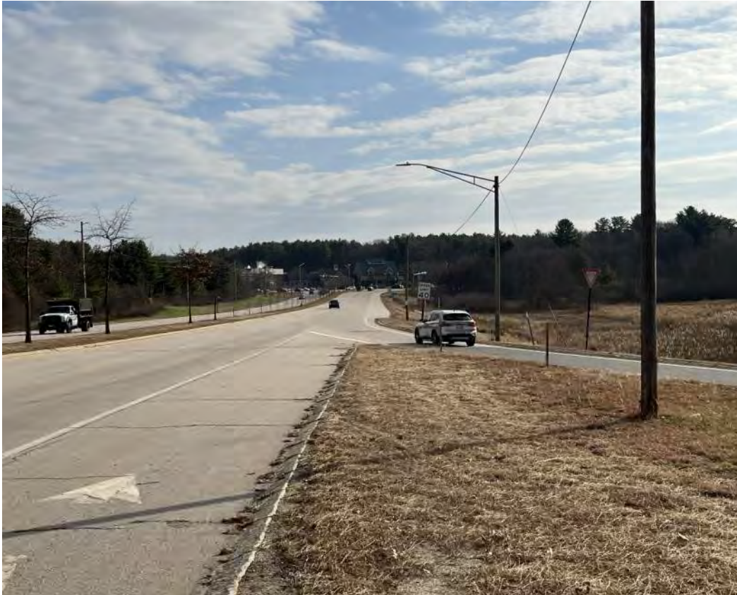
Photo 3: Slip Ramp Intersection from Spur Road (November 2022)
