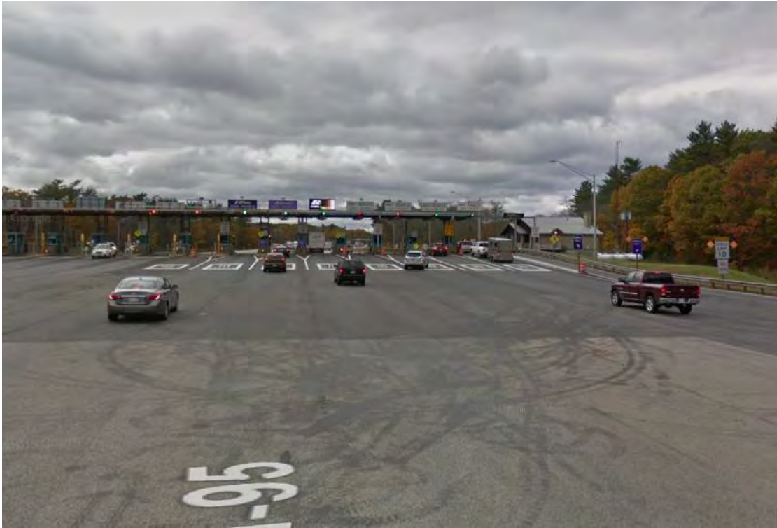
Photo 4: SB Toll Plaza (2018)
