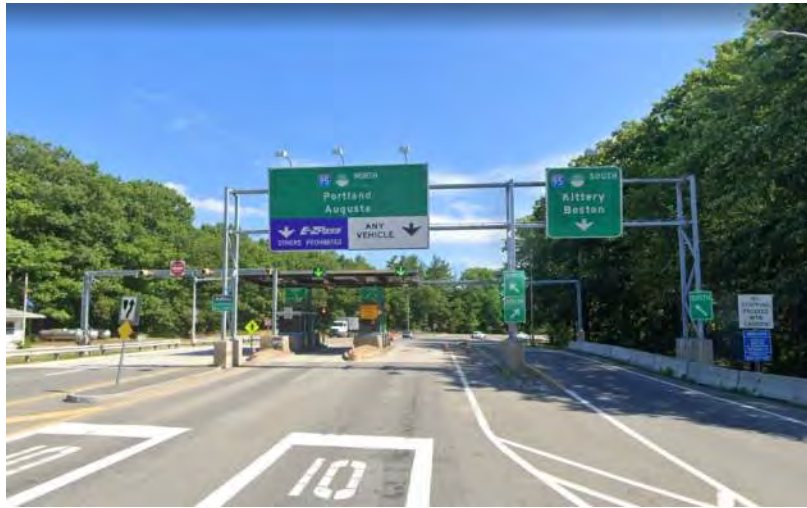
Photo 1: HCL 66 – Exit 19 Plaza Segment
