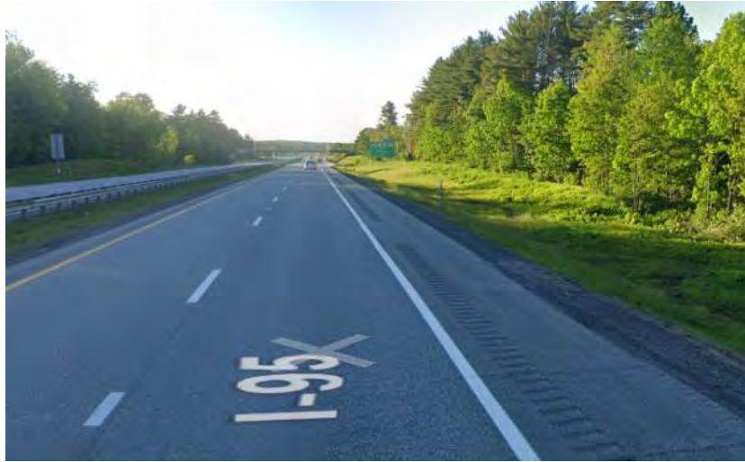
Photo 1: South of Exit 63 Off Ramp (2019)
