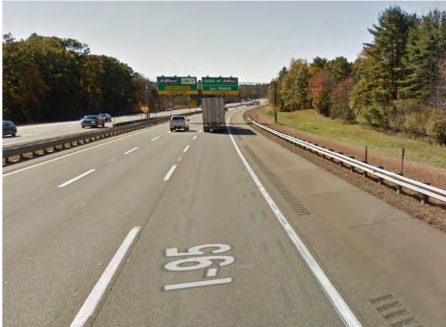
Photo 5: North of SB Toll Plaza
