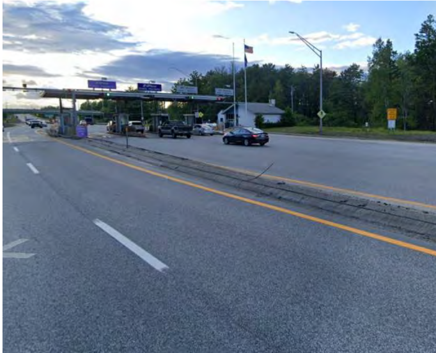
Photo 1: Exit 45 On Ramp Toll Plaza (2021)
