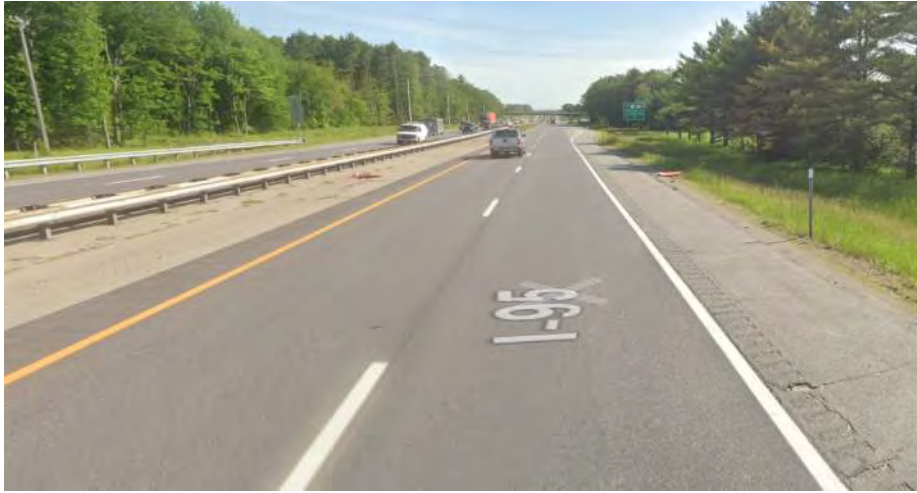
Photo 1: Exit 48 Southbound Approach (2019)
