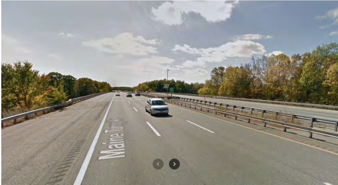
Photo 1: Mainline over Saco River
