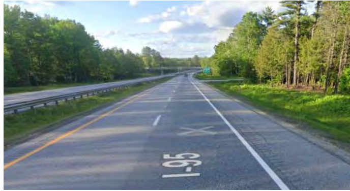
Photo 1: I-95 NB Near Poland Springs Bridge (2019)
