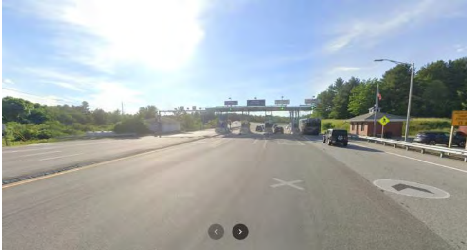
Photo 2: Exit 32 Plaza Ramps
