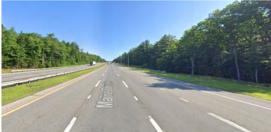
Photo 1: Exit 19 Northbound Mainline and NB On Merge
