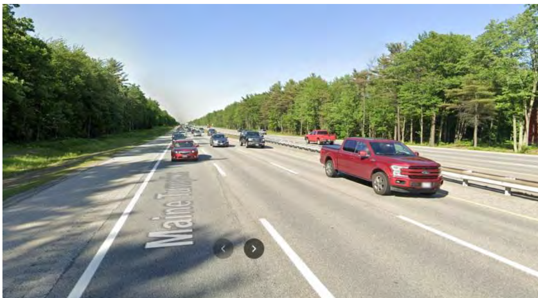
Photo 1: Just Prior to Exit 36 SB Off Ramp
