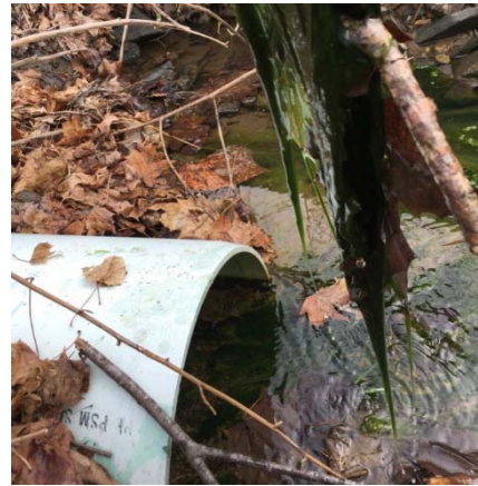
This outfall is partially submerged and a clean catch of its discharge is not possible. If tidal influences are strong, wait until low tide to sample. Additional options include: sampling upstream structures or using sand bags around the outfall to prevent contamination from backflow.
