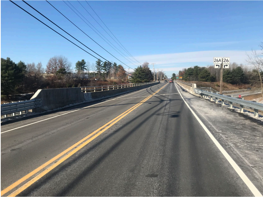
Shaker Road Bridge with surface pavement and finish striping.
