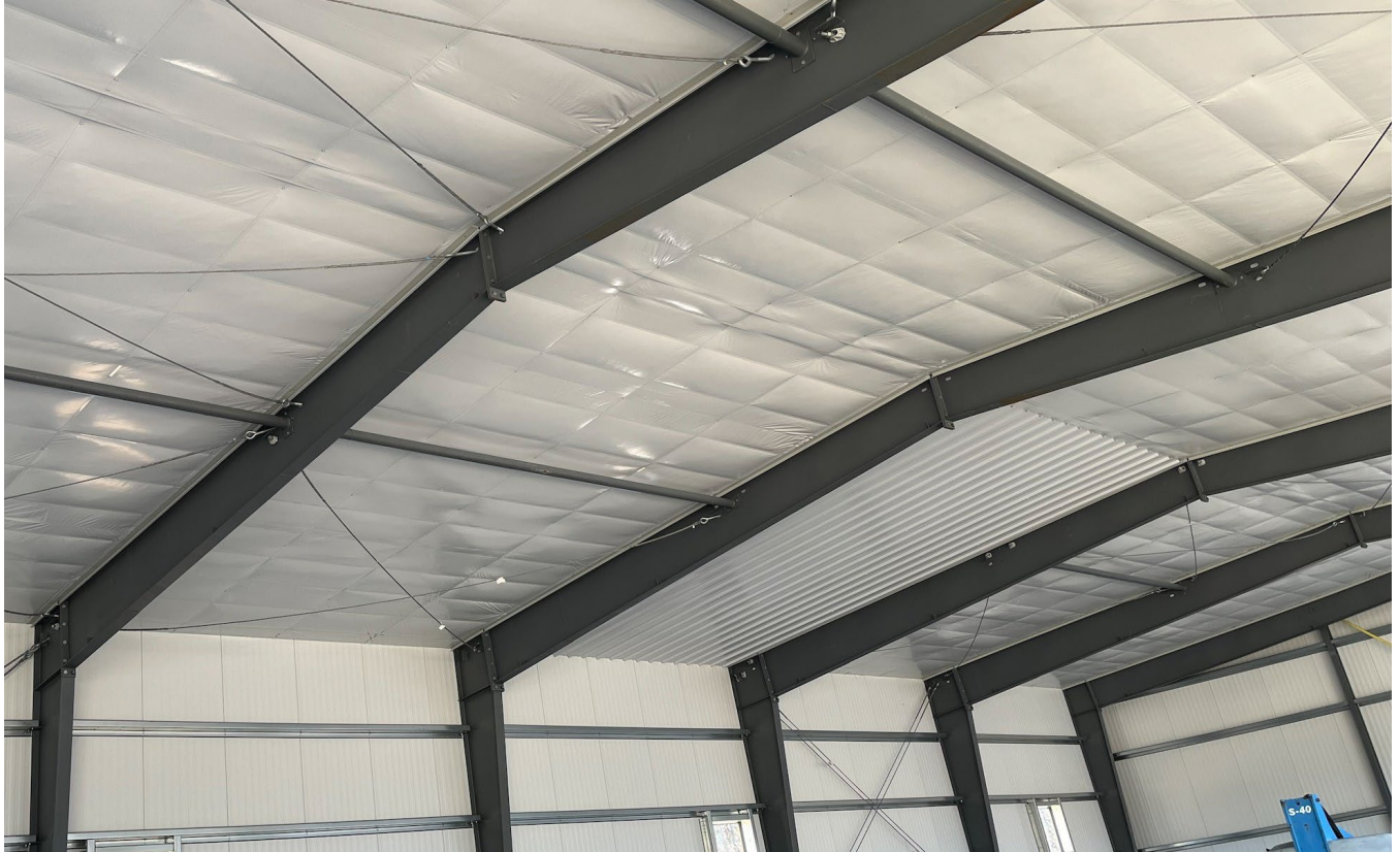
Looking east at the liner panels that cover the roof insulation
