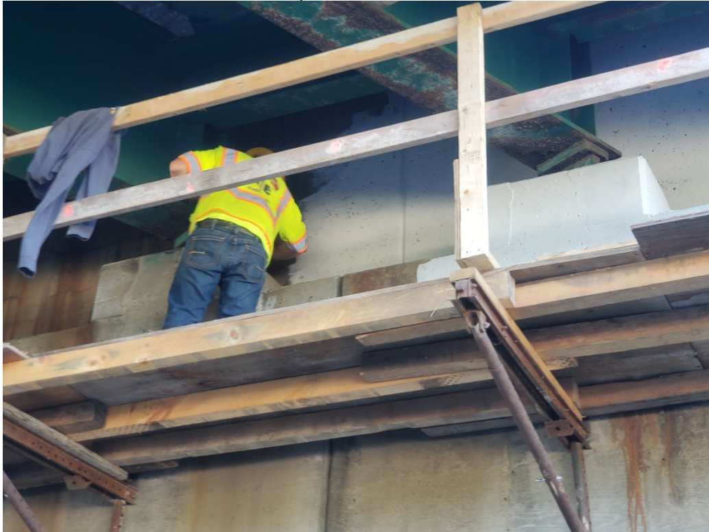
A worker applying pigmented coating to abutment at Route 236.
