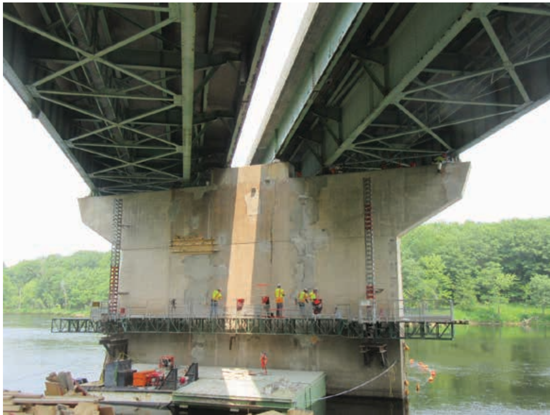
Androscoggin River Bridge Pier Rehabilitation, July 2019.
