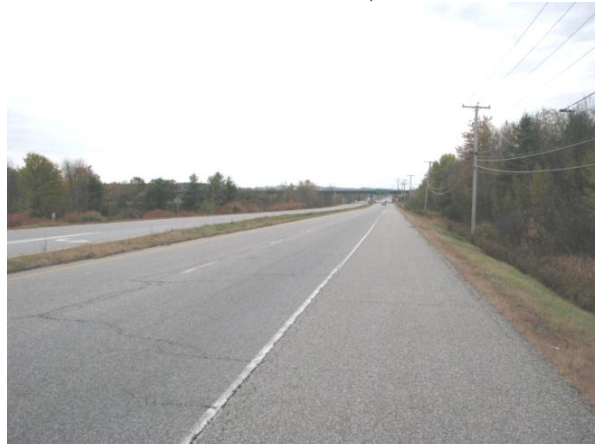
Figure 22 – Danville Corner Road/Beech Hill Road intersection looking south toward Turnpike
