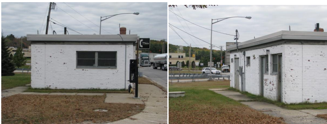
Figure 17 – Old toll building at Exit 75
