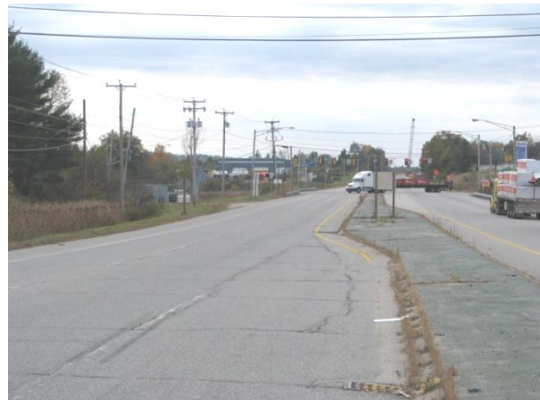
Figure 24 – Looking south toward the intersection with Kitty Hawk Ave.
