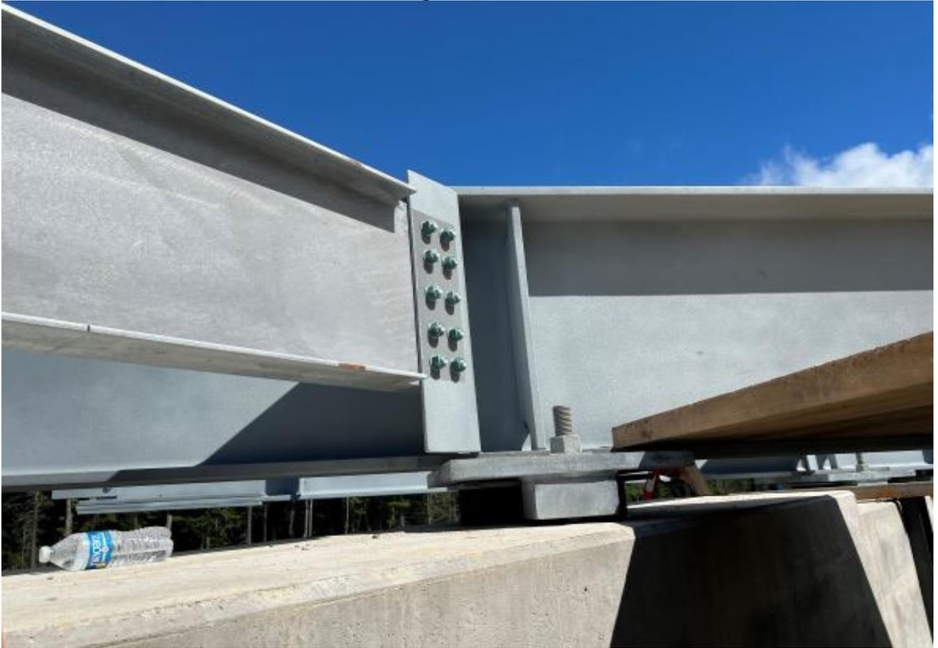
Looking north at pier 2, shown is the new bearing and girders for the Route 197 bridge.
