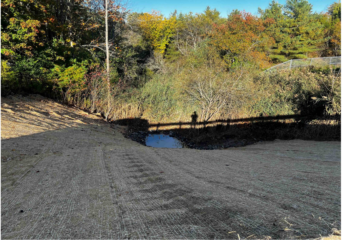
One of the deeper drainage repairs at Exit 52, southbound entering.
