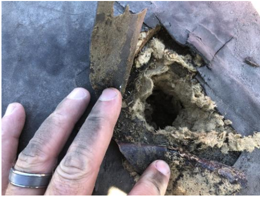
Figure 1: Roof Sampling
