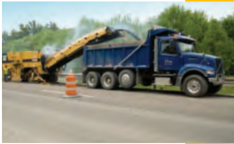
Turnpike contractors recycle pavement to reduce truck trips and costs.
