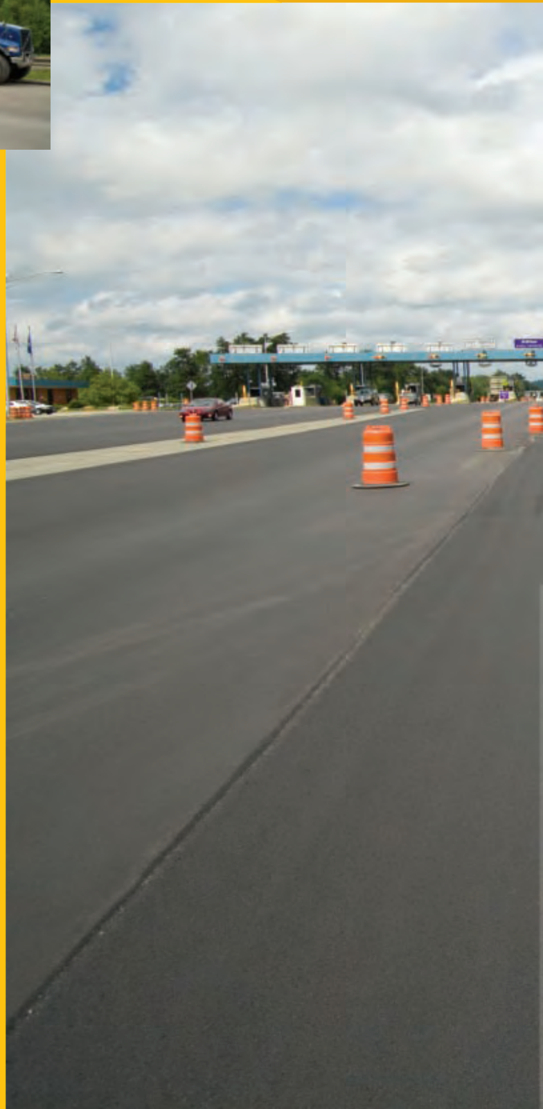
Turnpike contractors recycle pavement to reduce truck trips and costs.
