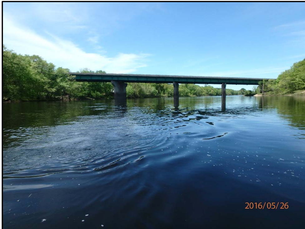
Photo 1 – South Elevation (Looking North)
