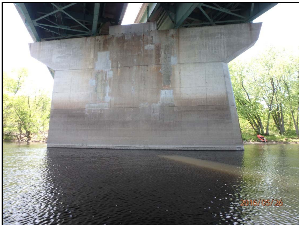
Photo 2 – Typical Pier Configuration (Pier 2 Shown, Looking West)
