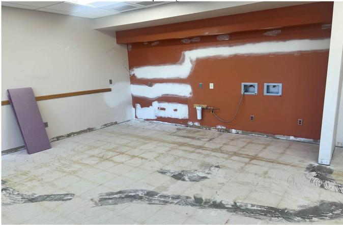
The first floor where the old kitchen used to be. The contractor is making repairs and updates before installing a new floor, cabinets, and countertops.
