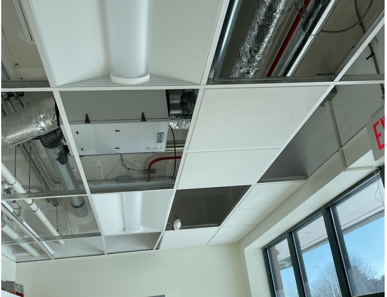
The northbound administration building ceiling tiles being installed.
