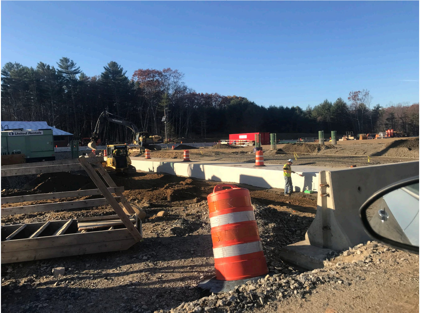
Contractor backfilling the tunnel, looking north.
