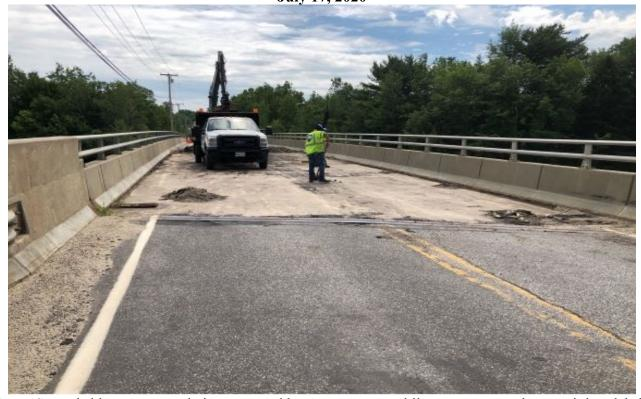
Grove Street bridge pavement being removed by an excavator while crews sweep the remaining debris.
