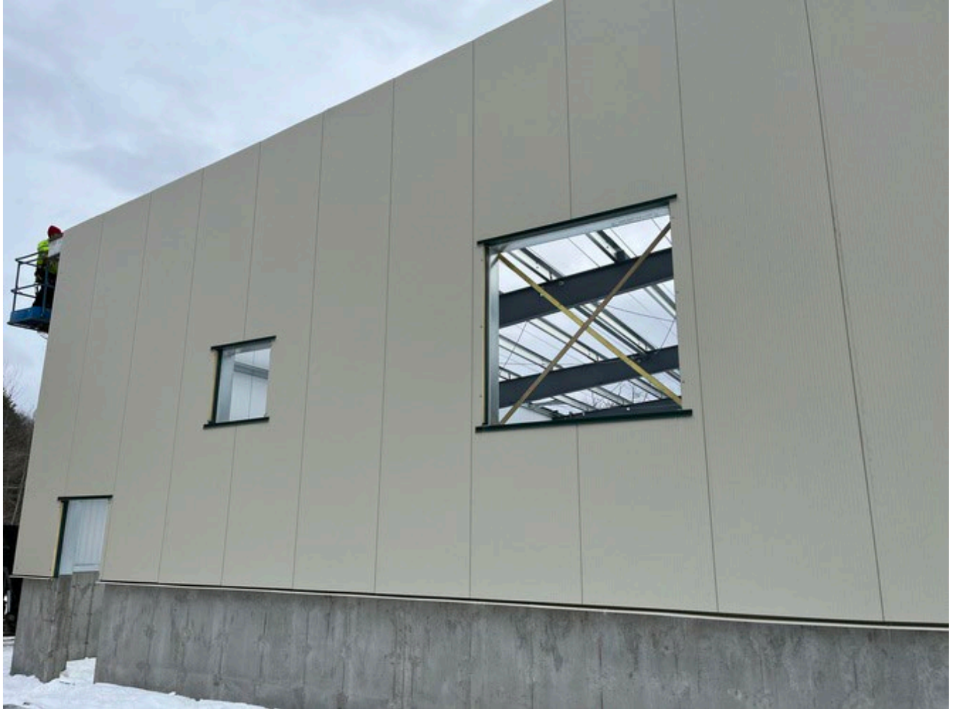
West side of the building without the roof system in place.
