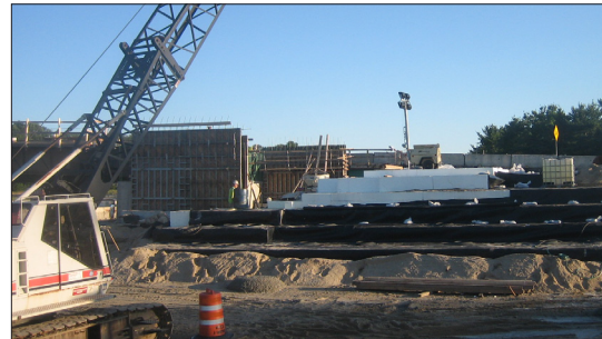
REPLACEMENT OF THE INTERCHANGE 48 BRIDGE
