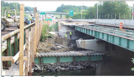
THE PRESUMPSCOT RIVER BRIDGE IS SCHEDULED FOR SUBSTANTIAL COMPLETION IN NOVEMBER 2011
