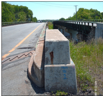
LISBON STREET BRIDGE PRIOR TO 2009-2011 RECONSTRUCTION
