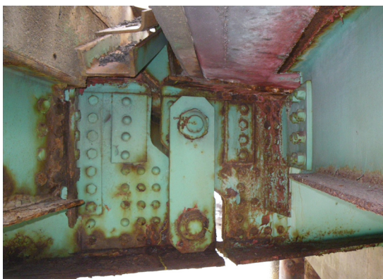
YORK RIVER BRIDGE PIN AND HANGER ASSEMBLIES
