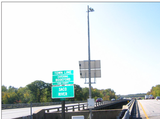
A RWIS WAS INSTALLED ADJACENT TO THE SACO RIVER BRIDGE OVERPASS
