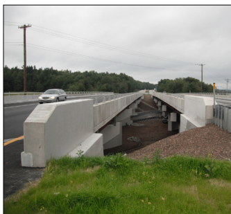
LISBON STREET BRIDGE AFTER THE COMPLETION OF CONSTRUCTION
