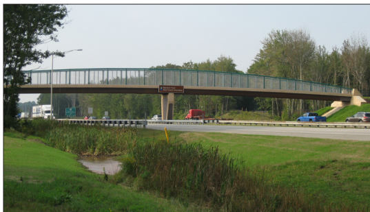
EASTERN TRAIL PEDESTRIAN BRIDGE CROSSING THE MAINE TURNPIKE
