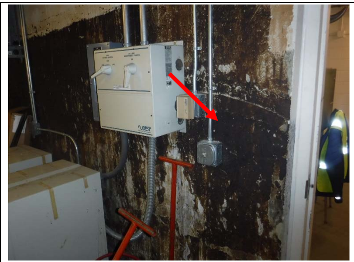
7. ACBM damp proof coating on perimeter foundation of original building. Photo shows exposed portion in lower level of Administration Building.
