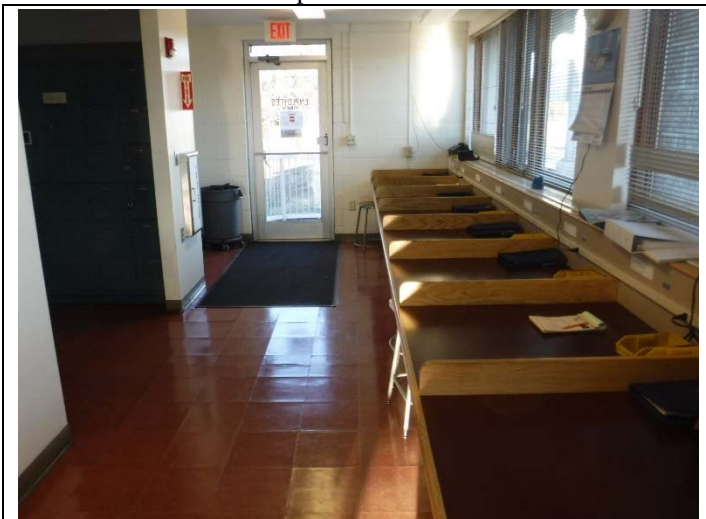
5. Typical interior of Administration Building with asbestos containing gypsum joint compound.
