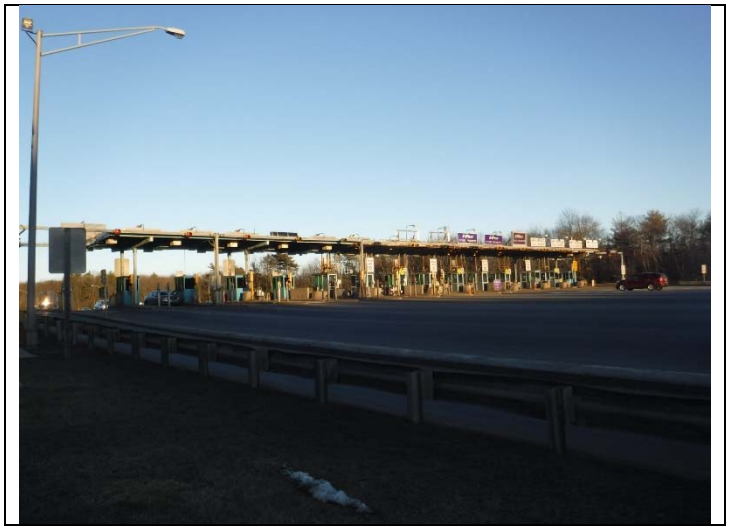
2. Toll Booths and Canopy
