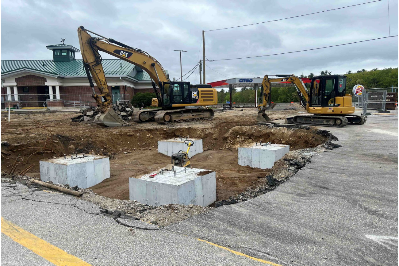
Looking north at the diesel canopy column foundations
