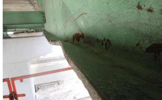
DUTTON HILL ROAD UNDERPASS, MILE 59.9
