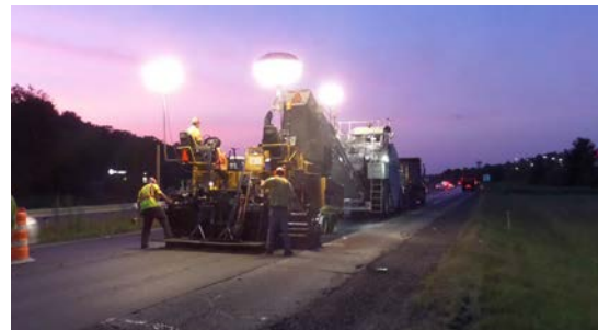
PAVEMENT REHABILITATION, MM 102.6 TO MM 109.1
