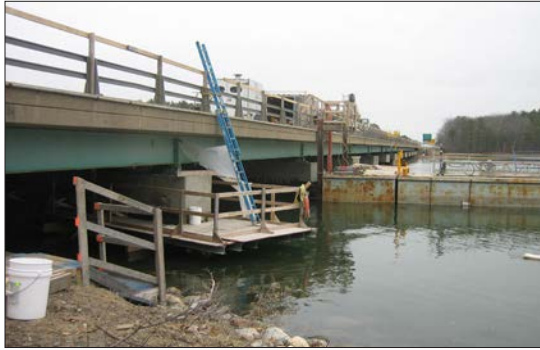
YORK RIVER OVERPASS, MILE 5.2
