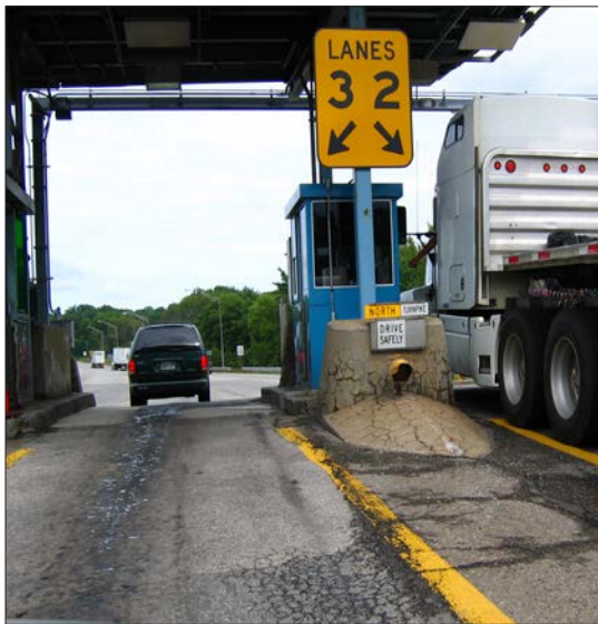
EXISTING YORK TOLL PLAZA - CONSTRUCTED IN 1969
