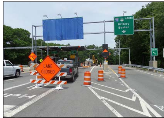
EXIT 19 TOLL PLAZA
