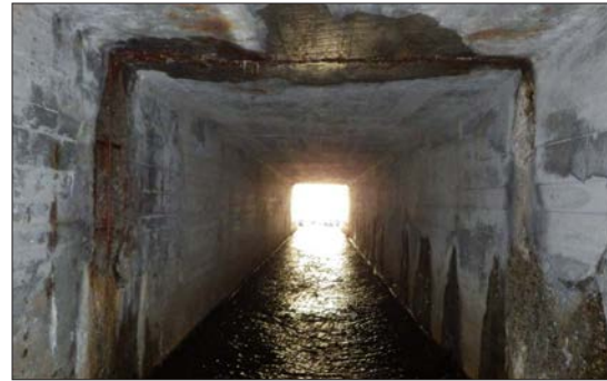
JOSIAS RIVER BOX CULVERT, MILE 11.8
