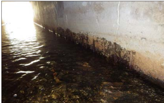
CAPE NEDDICK RIVER BOX CULVERT, MILE 9.6
