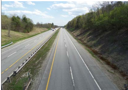
Mile 53.4, Looking South (After)
