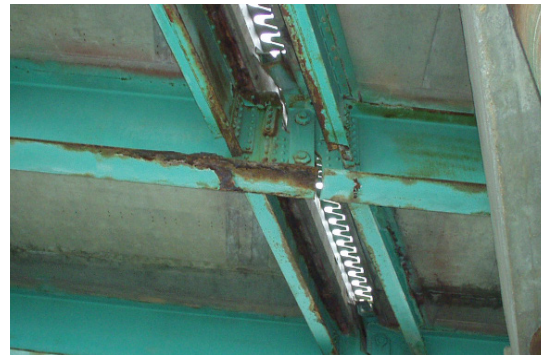
PIN-AND-HANGER ASSEMBLY UNDER A FINGER JOINT AT THE YORK RIVER BRIDGE
