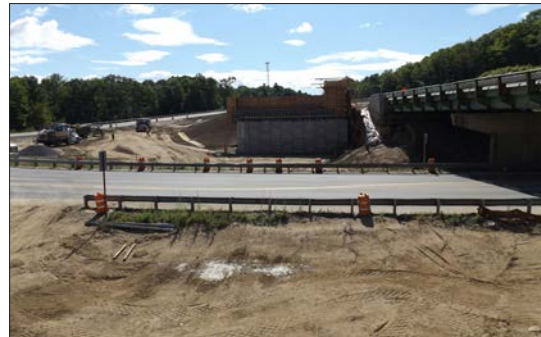
NEW LEWISTON BRIDGE UNDER CONSTRUCTION, MILE 80.3
