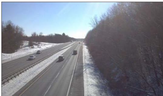
Mile 53.4, Looking South (Before)
