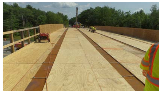
LUNTS HILL ROAD UNDER CONSTRUCTION, MILE 99.0
